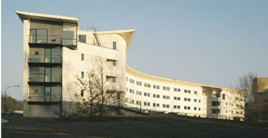
Figura 14 – Foto externa do Constable Terrace, University of East Anglia, Norwich, Reino Unido.
